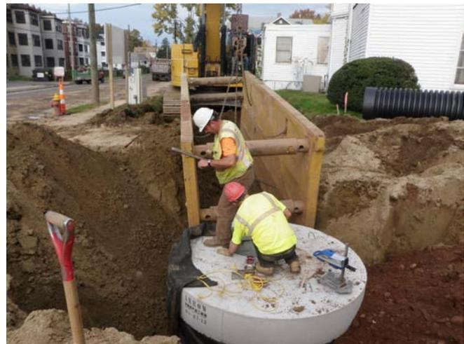
DTC's geotechnical engineering consultant, Comprehensive Environmental Inc., characterized the subsurface soil conditions as soft, low-plasticity clay and silt. None of the native soil would be suitable for refilling the trench due to compaction concerns. Trench refill with bankrun gravel as an alternative to native clay soil created a new problem. The increased weight of gravel when compared to the native clay soil was expected to induce pipe settlement on the magnitude of 1 to 3 inches.
